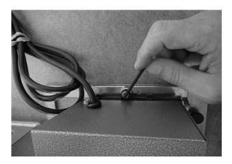
Photo 4. Install Shoulder Bolt
